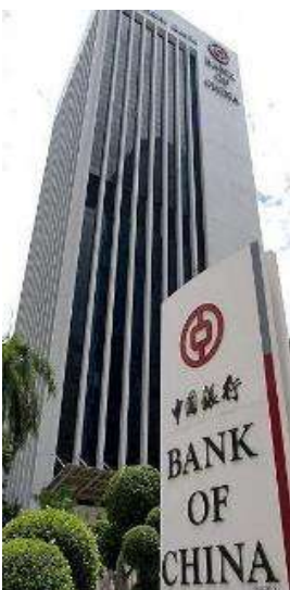
Bank of China, Ampang
