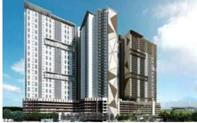
Platinum OUG Residence
