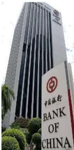
Bank of China, Ampang
