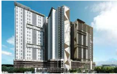
Platinum OUG Residence
